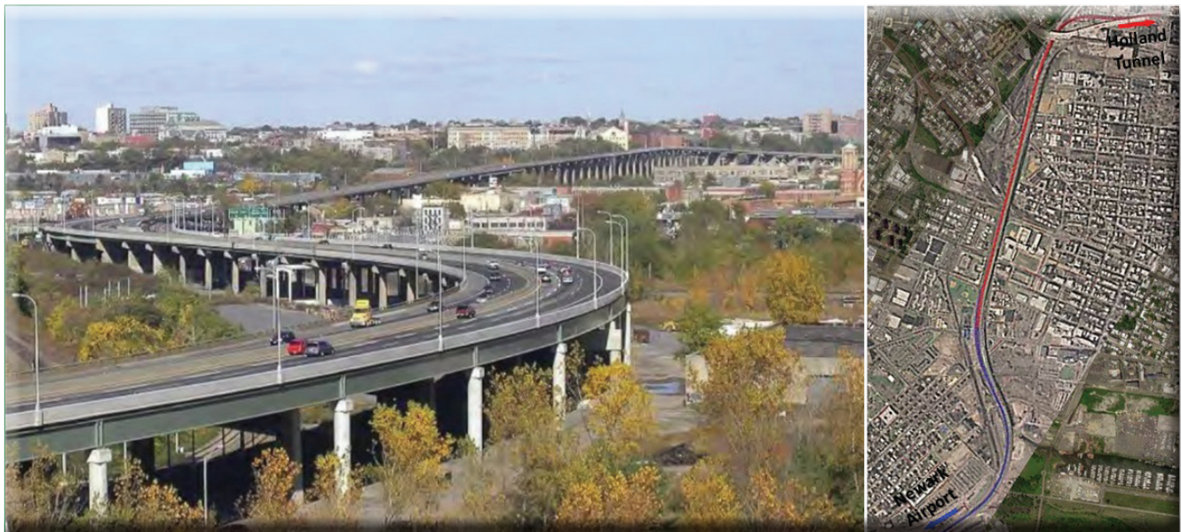
Figure 1. Bridge Overview for Field Implementation
